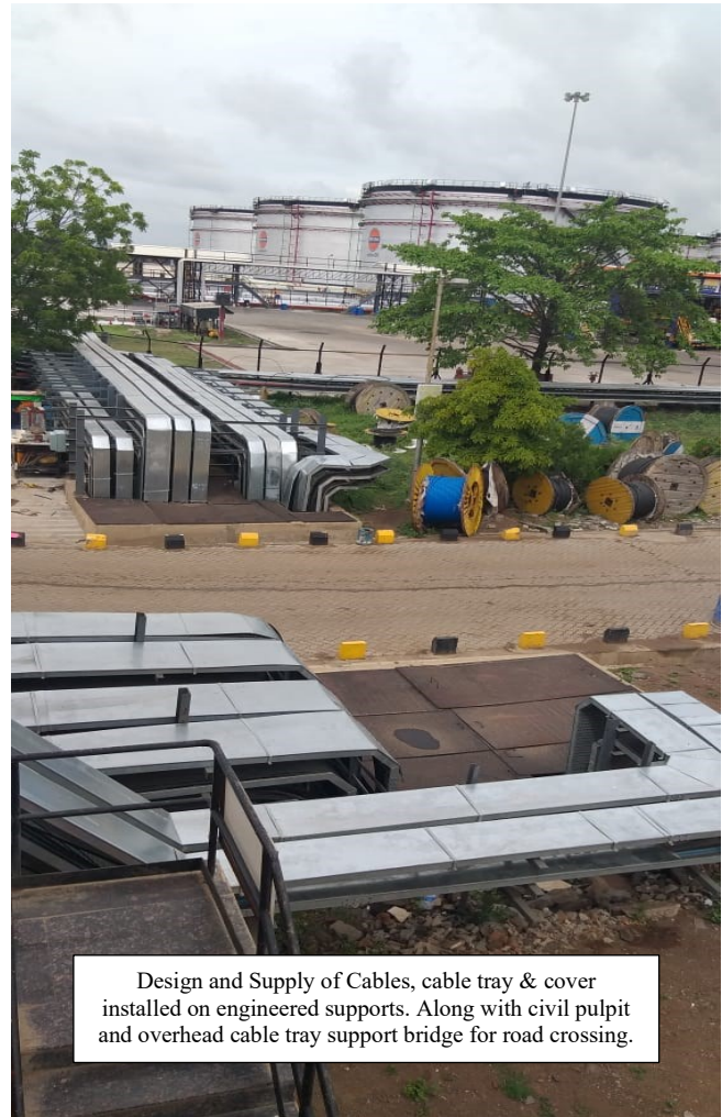
External Cabling System on Cable Trays
