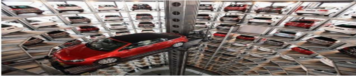
Fully Automated Parking System
