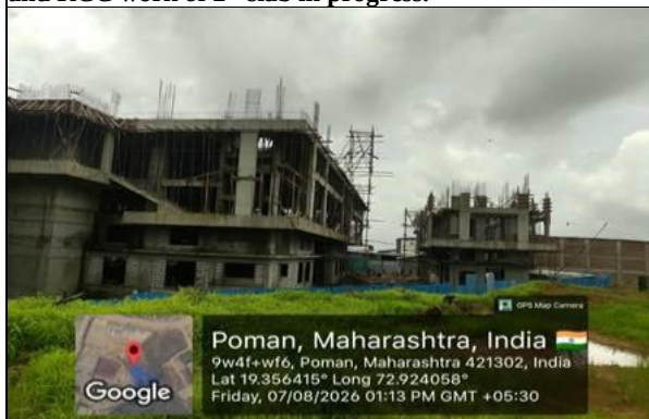
Top view of new manufacturing unit, depicting the construction of factory building after completion of 1 st slab and RCC work of 2 nd slab in progress.
