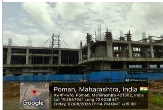
Side view of the factory building showing the front elevation of the factory building, including the RCC framework and boundary development works.
