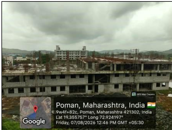
Top view of new manufacturing unit, depicting the construction of factory building after completion of 1 st slab and RCC work of 2 nd slab in progress.
