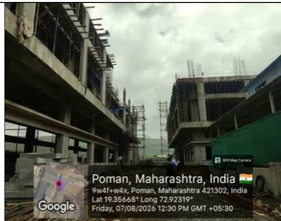
External view of the factory building showing the construction area and RCC structural framework.
